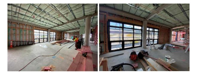
Internally, we continue to progress with the timber framing and services 1<sup>st</sup> fix (Cabling, pipework etc) installations on Levels 1 & 2. Plasterboard linings commenced this week to enable us to measure for the Hydration Station cabinetry.
